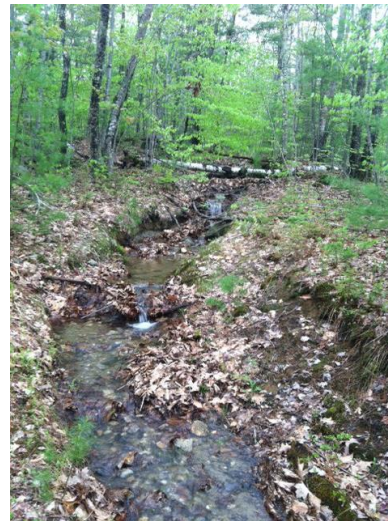
What appears to be a stream is a heavily eroded woods road that must be restored as a condition of the grant that paid for most of the property.
