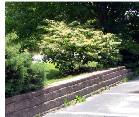
fig 8-3: Unbeveled Segmental Retaining Wall (SRW)
