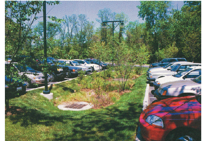
figs 5-2 & 5-3: Parking Integration into Natural Landscape; Stormwater Bioretention
