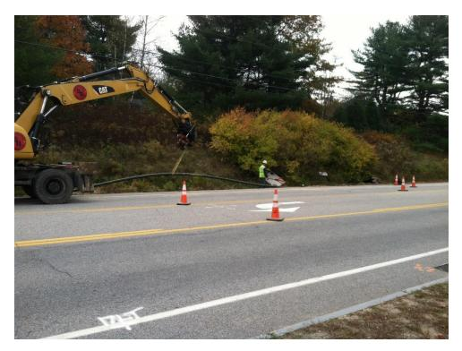
A work crew from Shaw Brothers Construction, contracted by Summit Natural Gas, is laying the gas main into a trench. This is near the southern end of the Route One Redevelopment Project work zone, just north of the intersection with Route 88.
