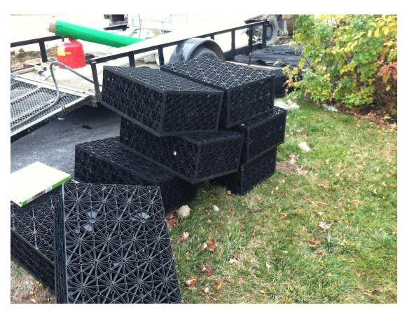
Next, these devices – called underdrains - are installed. They're basically plastic cages that facilitate collection of stormwater. More geotextiles are installed, then a layer of stone, and then a special biofiltration media is packed in. Crushed stone is placed atop this – followed, ultimately, by a layer of hardwood mulch and specially selected plantings. The result is cleaner stormwater runoff and an aesthetically appealing appearance.
