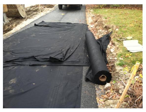
A biofilter starts with a rather deep hole, adjacent to a storm drain which collects street runoff. The hole is lined with several layers of geotextile, such as this...
