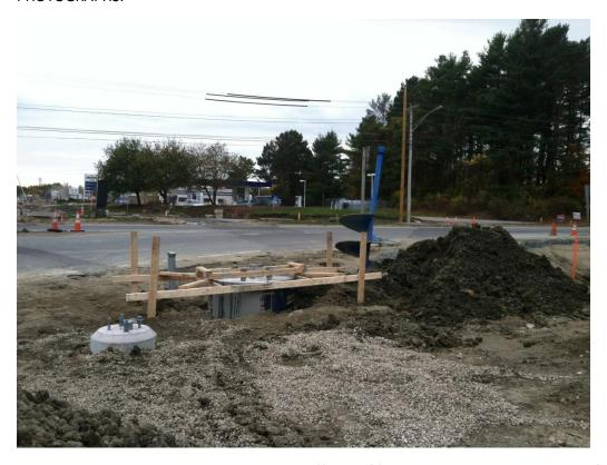
Looking south across Bucknam Road, we see (from left) a street lighting base; the base for a traffic signal pole, and the massive auger that dug the hole for it. This base was installed on 10/27; the concrete is still curing.
