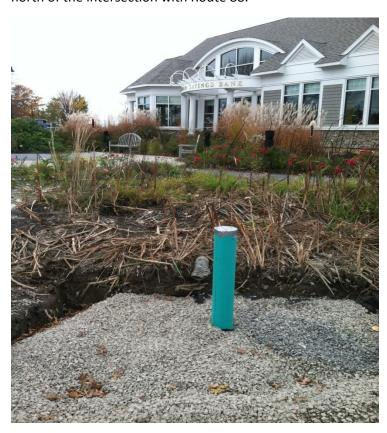
So what does a biofilter look like? Here's a nearly-completed one at the corner of Clearwater Drive, near the Gorham Savings Bank. Ultimately, the pipe will be cut down, the top will be mulched and vegetation will be installed. But there's much more than meets the eye. See below.
