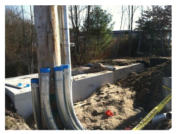
Here we see risers under construction on the east side of Route One, just north of the Irving Car Wash. The concrete structures in the background are utilities manholes. This location marks the north end of the project zone; from here, utilities emerge from the underground duct bank and resume overhead passage. Similar installations are just to the south of F. O. Bailey, towards the southern end of the zone.
