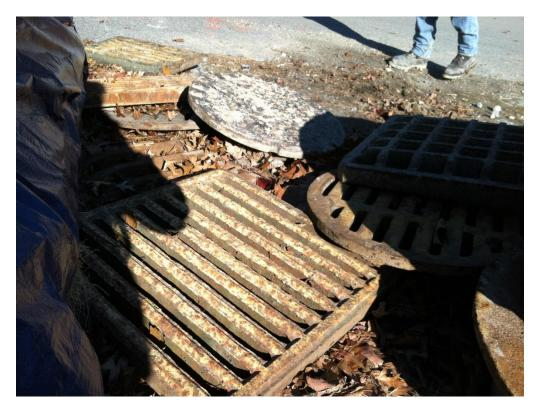
Here's an old catch basin cover that was removed during construction. Notice how the parallel grating could easily capture a bicycle tire. Because bicycle safety was an important planning consideration...
