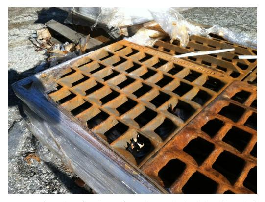
...covers in the roadway along the corridor are being replaced with these "cascading" grates. In addition to being much safer for bicyclists to ride over, the design of these grates allows a large volume of water to enter the catch basins with less turbulence.
