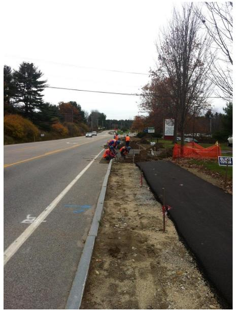
Looking south at the southerly end of the project, granite curb installers prepare and reset many of the radii curb that was previously removed.
