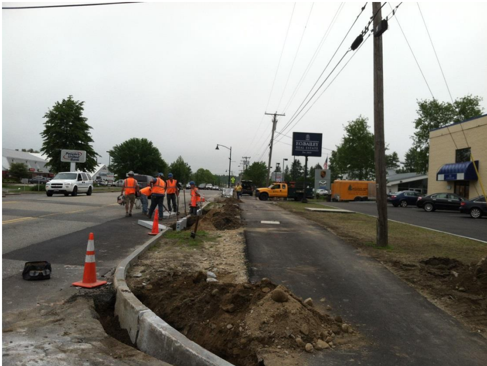
Looking north from the front of F.O. Bailey Antiquarians, we see a crew from Granite State Curbing installing new granite curbstone.
