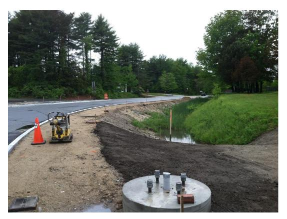
This view looks west on Bucknam Road, from the corner of Route One. In the foreground is the base for a traffic signal (expect to see those installed in a few weeks). At right, you can see grade work is complete for seeding. The sidewalk starting at left of frame is now graveled and graded, leading up to the Maine Medical Center campus across from the fire house.
