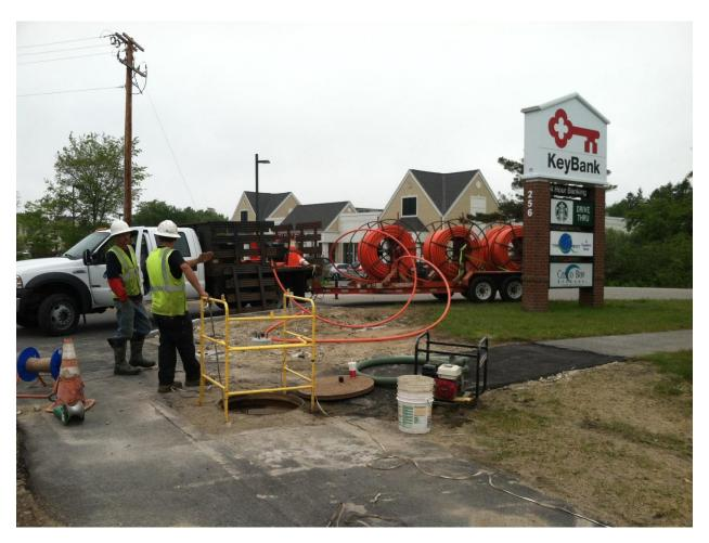
In this photo, we see what's called an "inner-duct." An inner-duct is essentially a conduit-within-a-conduit; it helps protect fiberoptic cable. Here, we see a subcontractor team for Oxford Networks in the process of installation. You may have noticed another crew today at the corner of Bucknam Road. This is the last major underground utility installation.
