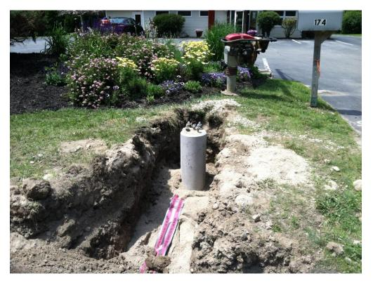
Here's a base fixture installed – with wiring already in place. This unit is just south of Waldo's, on the west side of Route One.
