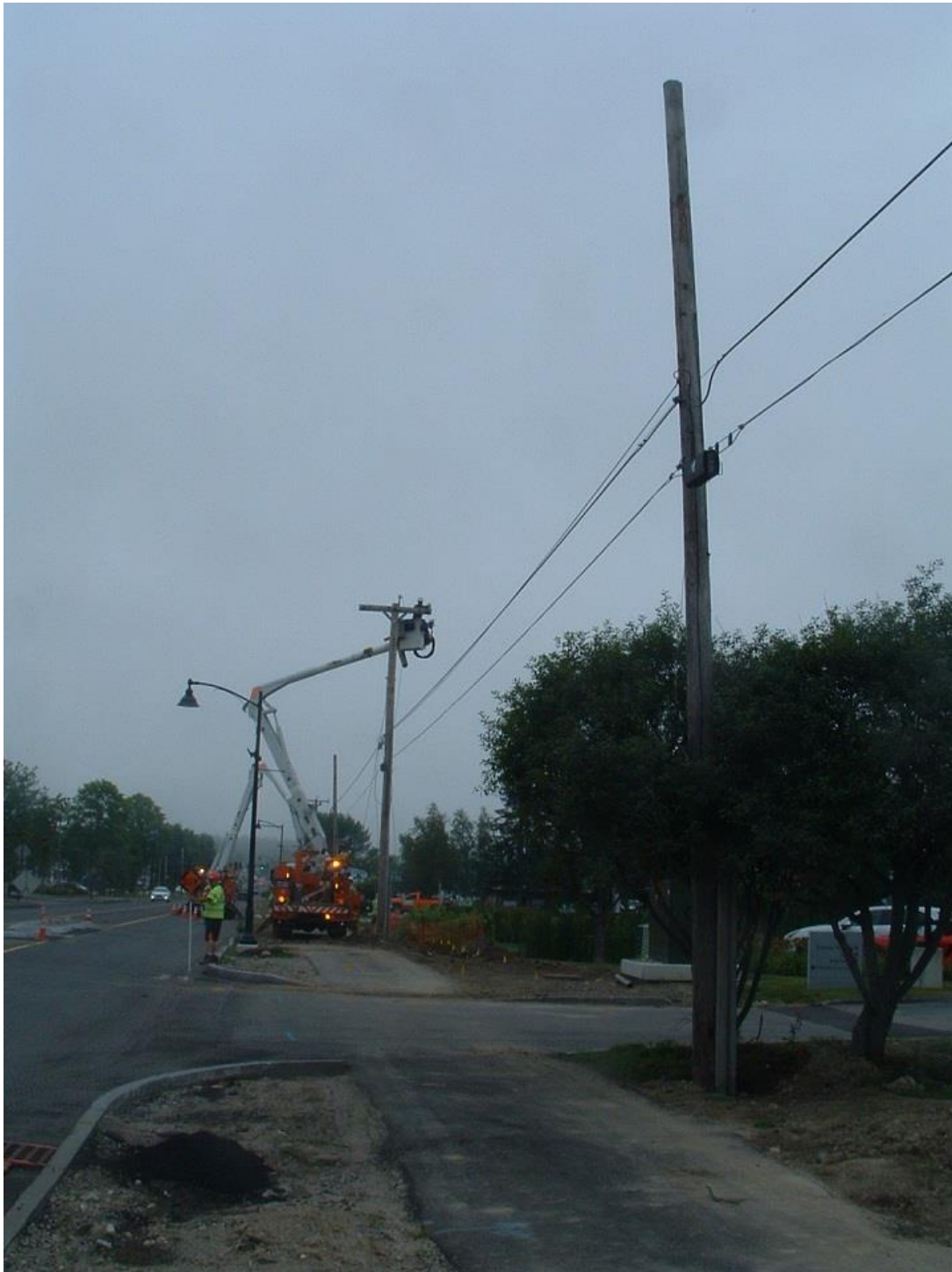
Here we see a crew from CMP removing overhead power lines. That's a fiber optic cable remaining on the poles; these should be removed shortly. Crews expect to start removing the utility poles this Thursday.
