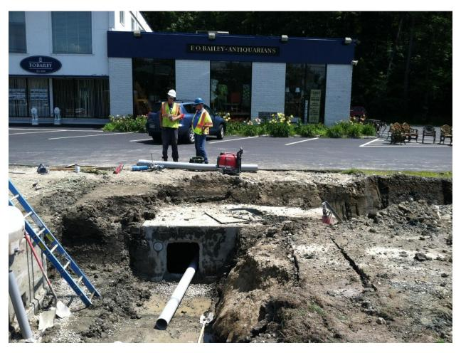
Construction workers in front of F.O. Bailey Antiquarians. In the center and left of frame are two newly installed manhole structures – one for electrical service, and one for other utilities.
