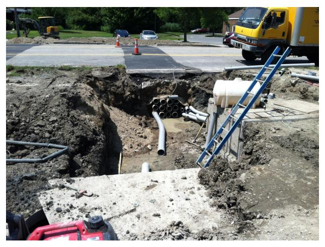
The crossing of Route One carrying electrical and utility conduits from the main duct bank on the west side of the road (across from F.O. Bailey Antiquarians). These conduits were installed overnight last week and the road cut, like all cuts made to date, has been re-paved, permitting smooth two-way flow of traffic.
