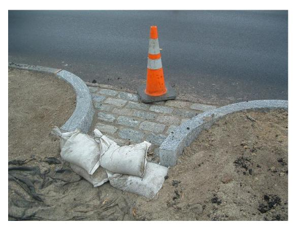
Here we see a nearly-completed biofilter entrance, freshly cobbled. In all but winter months, stormwater will be channeled into the biofilters by means of the granite curbstone. During the week of September 7, the biofilters will be finished with the addition of an attractive mix of shrubs and perennial grasses and flowers. The biofilters remove petroleum products and other pollutants from stormwater runoff, reducing the amount of pollutants reaching Casco Bay.
