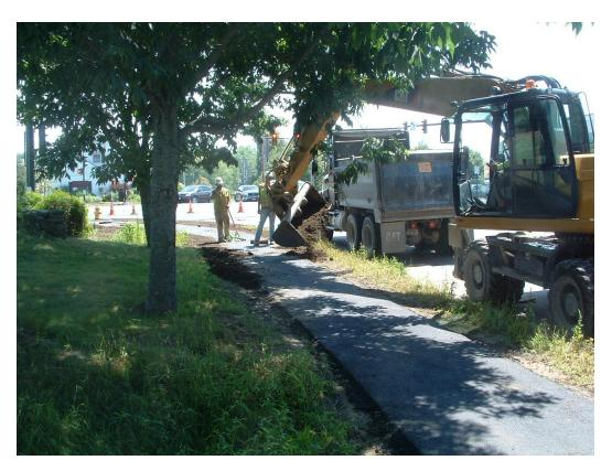
Here's a crew from Sargent Corp. working on landscaping on Depot Road, looking east. With finish-grade paving now in place, the crew is fine-tuning the loam grade in preparation for seeding.
