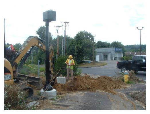
Here we see a crew installing one of the last pedestrian light bases. This is adjacent to the Leavitt and Sons Deli; the base casting couldn't be installed until a utility was removed. A handful of other light bases and pedestrian tactile warning strips are still to be installed.
