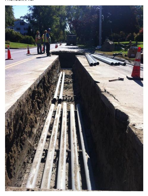
We're looking east on Depot Road, where Moulison North is installing underground communication conduits. These conduits will tie in to an existing 'sub-station' near Foreside Road which is owned by Fairpoint Communications.
