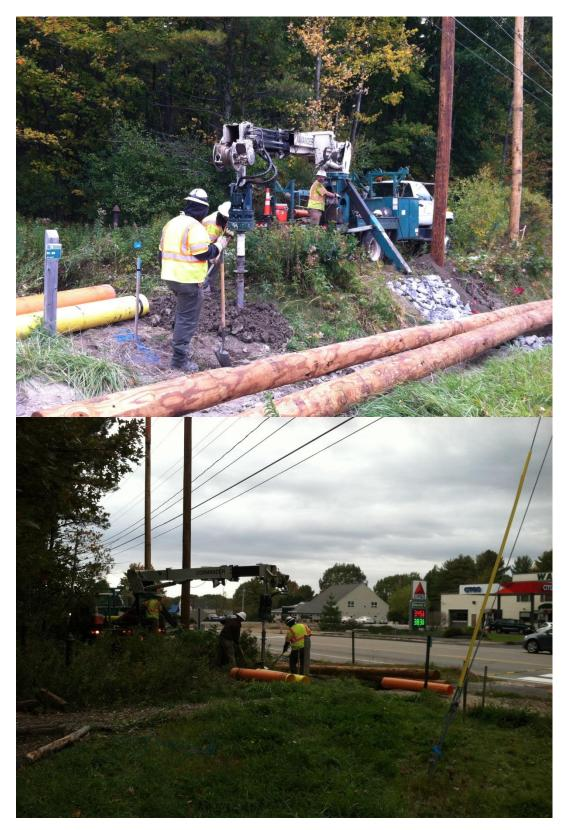
In these images – taken across the street from Waldo's and just south of F. O. Bailey Antiquarians – we see a crew from On Target (contracted by CMP) in the process of installing several permanent utility poles. Electrical and data service will "drop" from these poles, and feed the underground duct bank that will provide services to the majority of businesses in the project zone.
