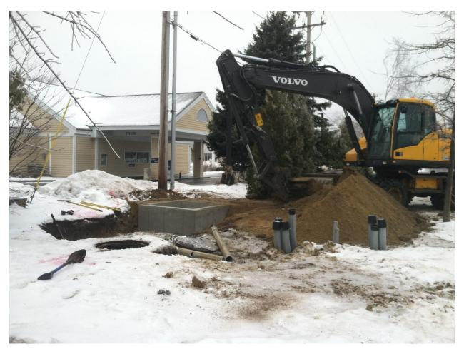
This is the final piece of major work by Moulison North – a spur of the duct bank (that's the Bath Savings Institution in the background). Once this work is completed, Moulison has a few manholes to raise and a small amount of electrical work remaining near Morong on the west side. After that? Expect cables to be pulled through the duct bank over the winter.
