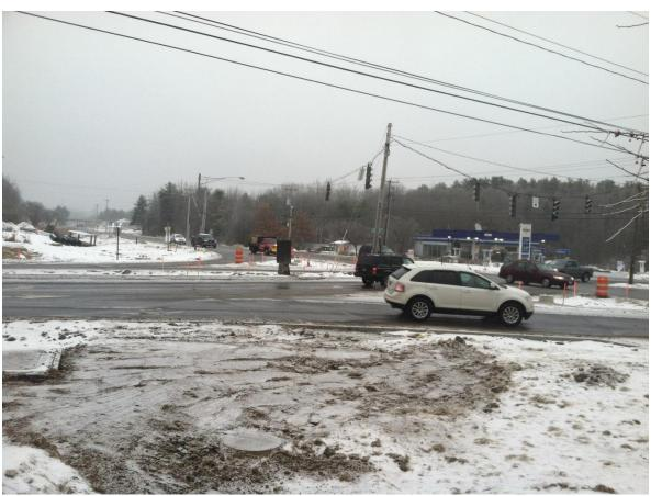
Here's the Bucknam Road intersection, looking northeast from in front of the Irving convenience store. The islands and road edges have been curbed. Stakes and barrels are in place to guide plow operators and cover bases for pedestrian lighting and signals.
