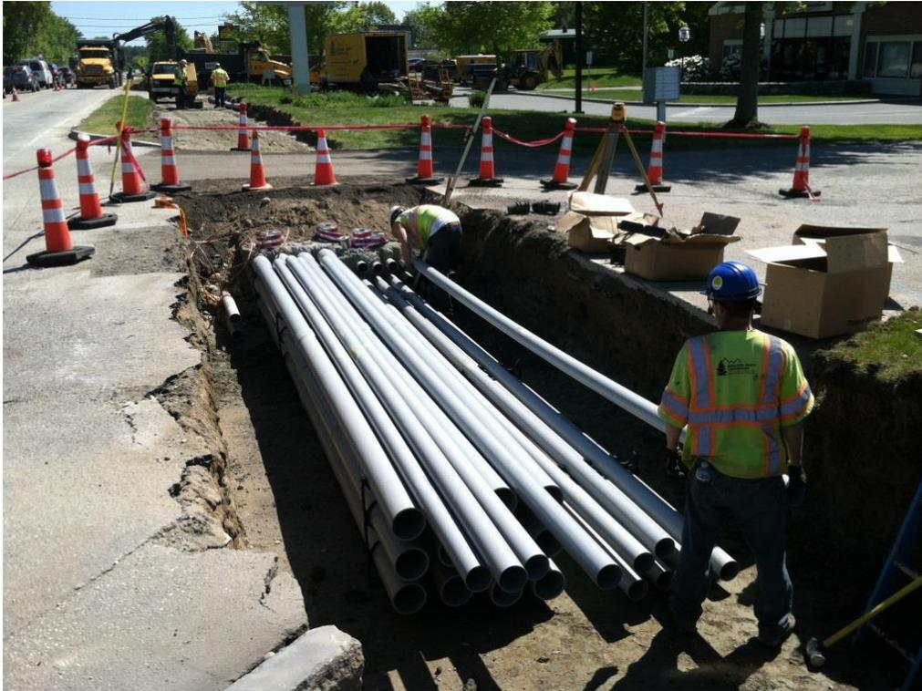
*In this photo, we see a crew from Moulison North Electrical Contractors installing the conduit bank. These lines will carry electrical, phone, and communication services. Once these lines are fully installed, energized, and connected with Route One businesses, overhead electrical and data lines will be removed, creating a much more attractive streetscape.*
