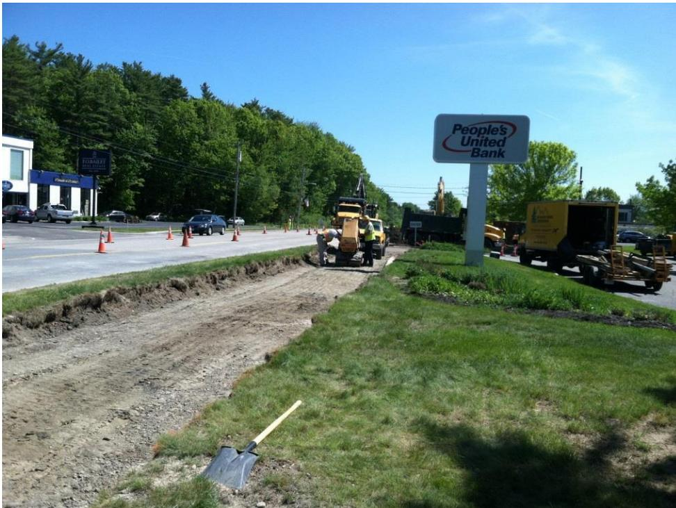
*Here, crews have buried the first sections of the communications conduit, and are grading and compacting the backfilled area so that the new sidewalk can be installed.*
