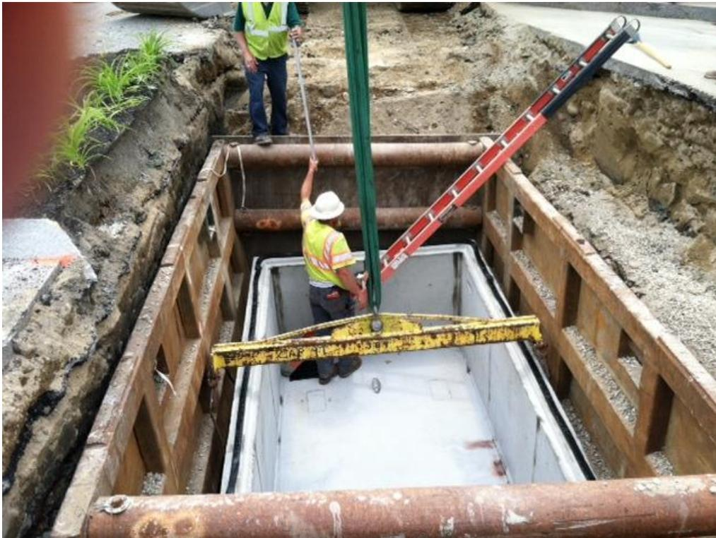
*The foreman descends into the bottom half and carefully checks for level. It is perfect, thanks to careful preparation before the hoist. The black strip (gasket) on top of the structure is installed to seal the top section to the bottom.*
