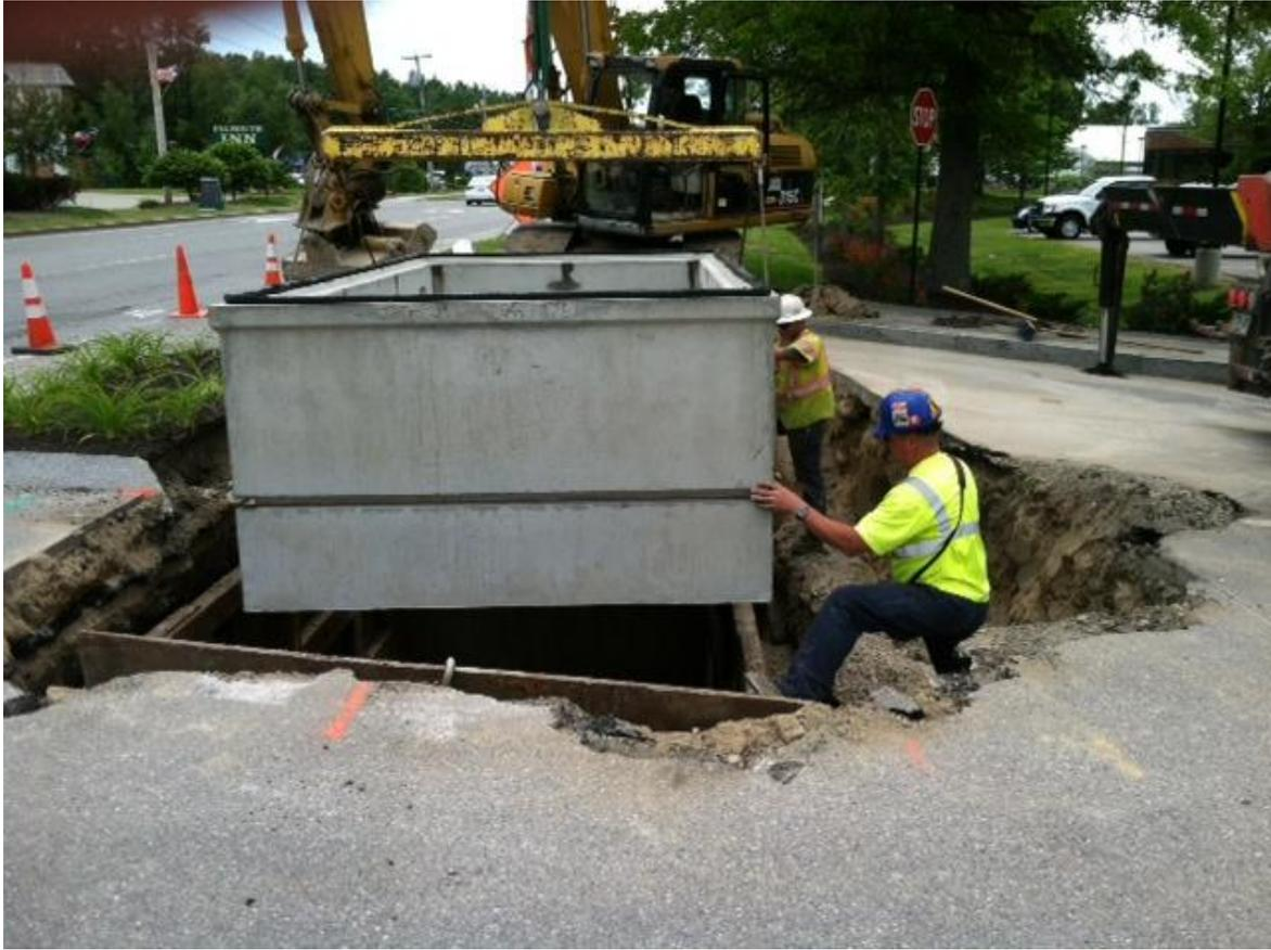
*The crew carefully aligns the structure over the pit and lowers it into place.*
