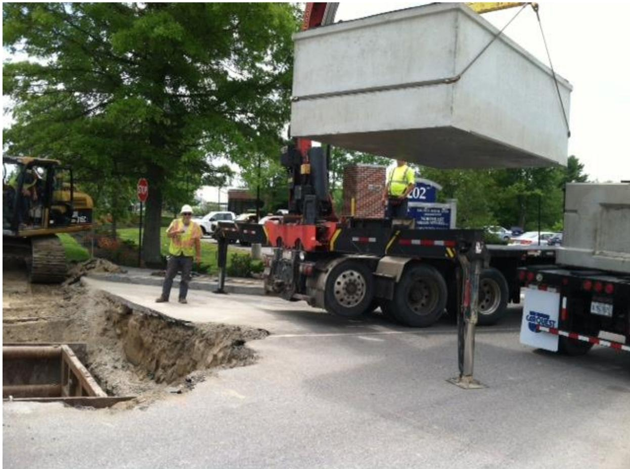
*The bottom half of the electrical manhole is lifted and carefully swung into position.*
