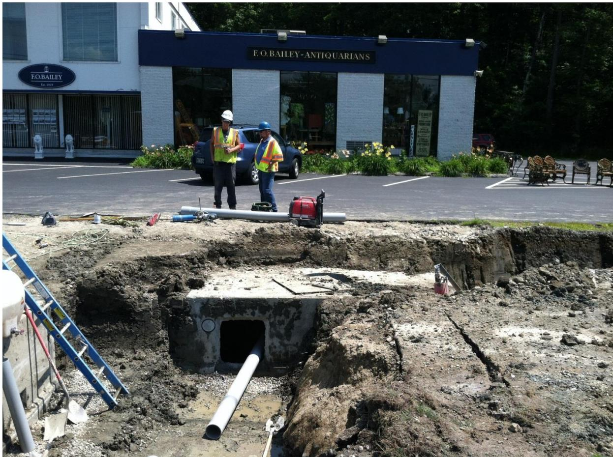
Construction workers in front of F.O. Bailey Antiquarians. In the center and left of frame are two newly installed manhole structures – one for electrical service, and one for other utilities.
