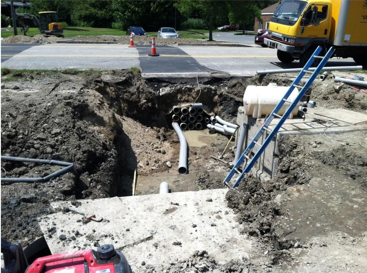
The crossing of Route One carrying electrical and utility conduits from the main duct bank on the west side of the road (across from F.O. Bailey Antiquarians). These conduits were installed overnight last week and the road cut, like all cuts made to date, has been re-paved, permitting smooth two-way flow of traffic.
