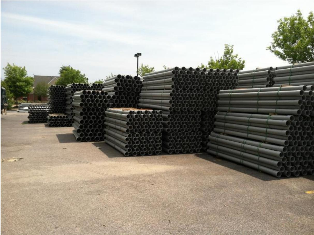
The conduit bank uses a LOT of plastic pipe – 20 miles or so, by the time the project is complete. Excavators dig a trench, then crews carefully install the pipes. A form is built around it, and then the conduits are embedded in concrete before backfilling. You may have noticed manhole structures along the way, too. Once the conduit bank is completed, utility companies will pull their lines through the conduits.
