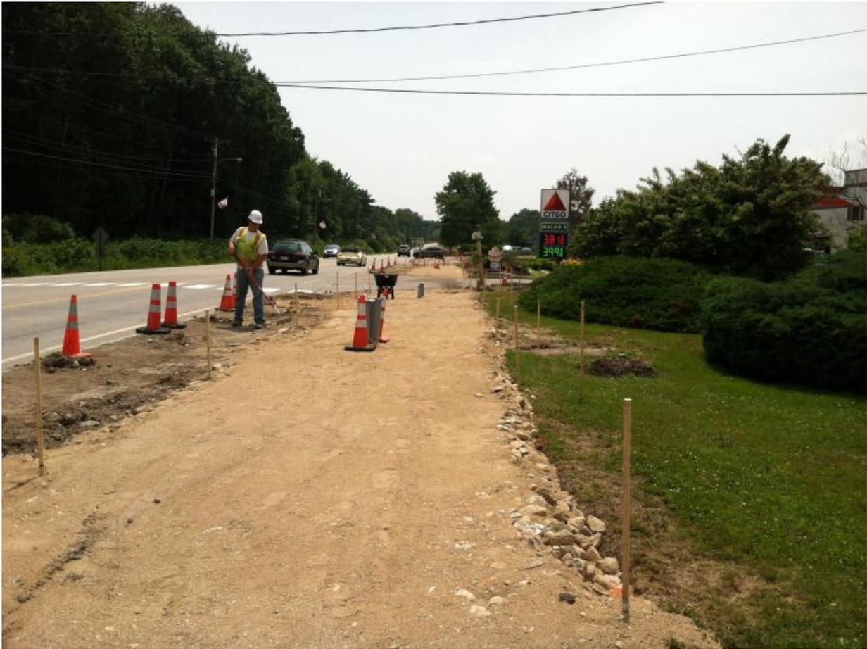
A worker puts final touches on grading of the sidewalk, readying it for paving later this week.
