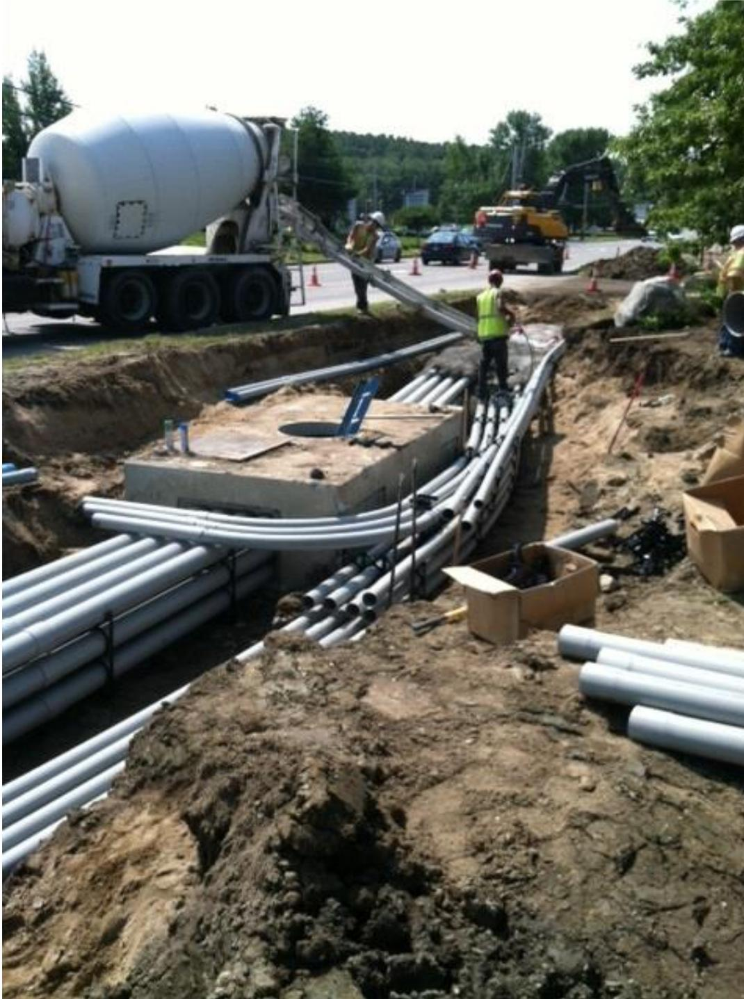
This shot was taken last Wednesday and shows an electrical manhole installation. Note that the conduits for power run through the manhole and conduits for other utilities (telecommunications) run outside of it. These conduits will enter utility-specific manholes in other locations. The conduits are encased in concrete, then backfilled with soil.
