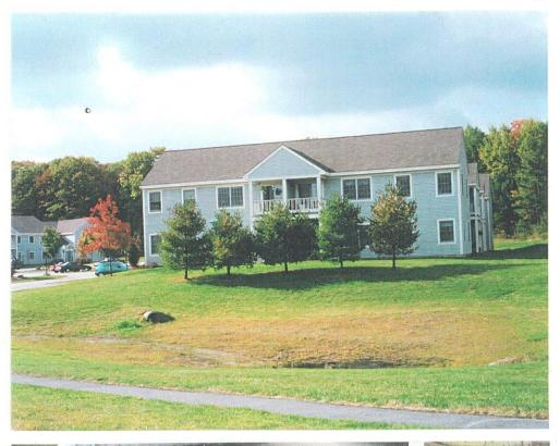
Standing water in the detention basin has apparently killed the grass below the 'ring'. Careful design and knowledge of soils and groundwater conditions are necessary to achieve a successful result. Wetland plantings in the basin may have been a better choice.
