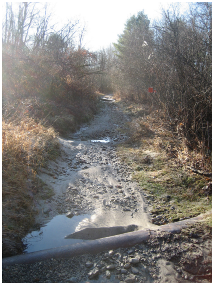
The CMP access road along the river is heavily washed out. It needs to be relocated.
