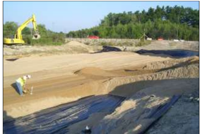
Installation of a large water quality sand filter at the Portland International Jetport.
