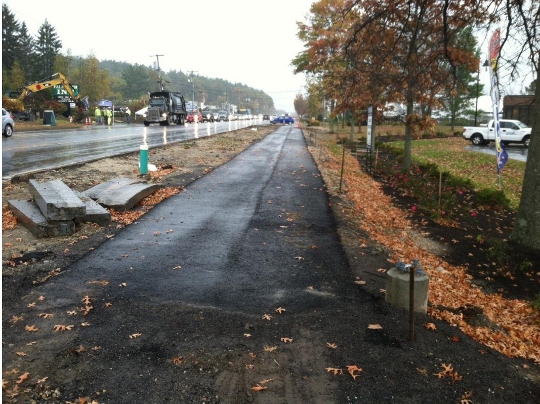
Looking south, from roughly in front of Orchid Thai, we see sidewalk and curbing. In the lower right of the frame, we see the base for a pedestrian walkway light pole.
