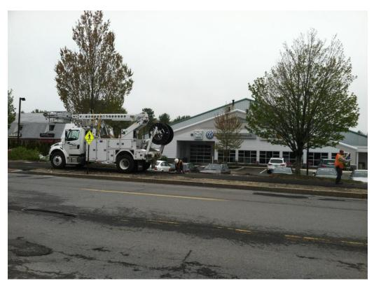
Fairpoint is still pulling fiber optic cable in various locations along the corridor. In this image, we see a crew wrapping up a pull through the duct bank crossing under Route One.
