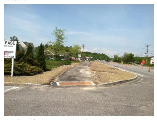
We're looking north from the entrance to the Shops at Falmouth (Staples, Ricetta's, Pet Quarters, etc.) This area has been backfilled with loam and hydro-seeded. Much of the west side of Route One has had similar work, and grade work on the east side is currently occurring.
