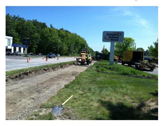
Here, crews have buried the first sections of the communications conduit, and are grading and compacting the backfilled area so that the new sidewalk can be installed.
