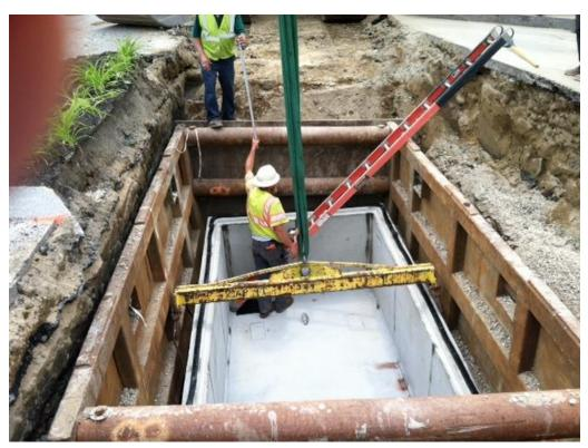
The foreman descends into the bottom half and carefully checks for level. It is perfect, thanks to careful preparation before the hoist. The black strip (gasket) on top of the structure is installed to seal the top section to the bottom.
