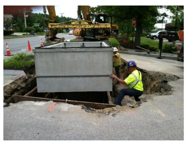
The crew carefully aligns the structure over the pit and lowers it into place.
