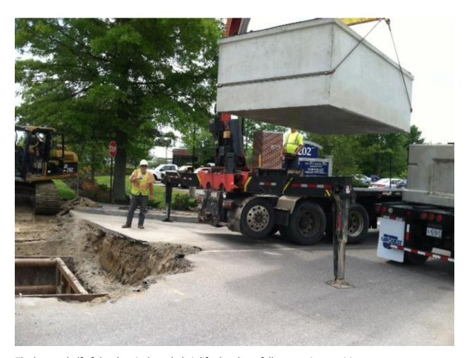
The bottom half of the electrical manhole is lifted and carefully swung into position.
