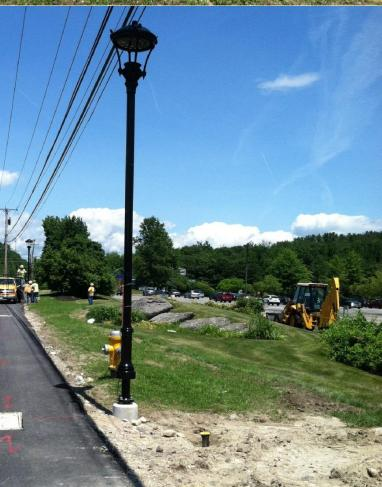
Here's one of the new sidewalk lights mounted to its pedestal. The decorative collar is tied above the base, awaiting an electrician to connect the wiring. The lighting element consists of a complex array of light emitting diodes (LEDs), ensuring long life and minimal power demand. You'll be able to see this fixture without all those overhead wires in a few weeks.
