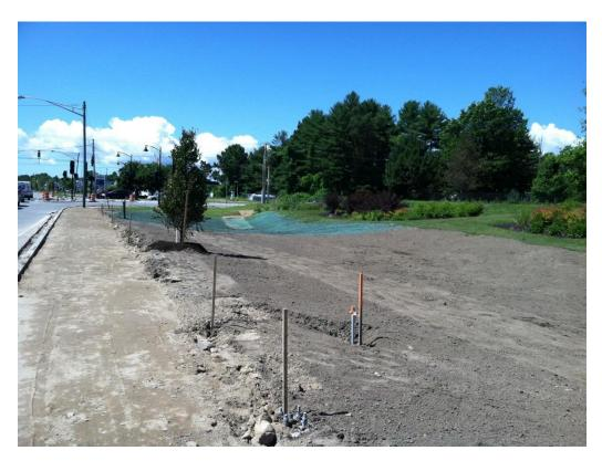
We're just north of Bucknam Road, looking south. The stormwater runoff requirements in front of the Norway Savings Bank were among the most complex along the entire corridor – and this is the last major area to be finish-graded. At left, you can see the sidewalk prepped for paving (which should happen tomorrow); at right, a newly planted tree, and an area that's been hydroseeded. The pipe sticking up center left will soon be a fire hydrant.
