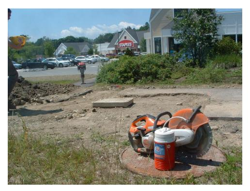
This is work in front of Olympia Sports and involves some finalization of electrical work. That's a quazite box (a junction box) in the center of the frame; just above it is a newly-placed foundation for one of the handful of pedestrian lights that are yet to be installed. The odd-looking device in the background is a compactor; soils must be well-compacted in advance of finish paving of the sidewalk, in order to ensure a durable surface.
