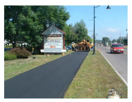
We're looking north along the west side. This is a crew laying down finish-grade asphalt on the sidewalk.
