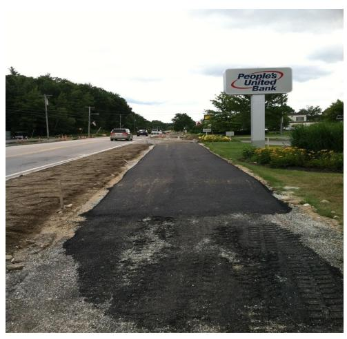
Base layers of sidewalk paving now reach from Waldo's almost to Morong's Service Center on the west side of Route One. Please note that this paving is not continuous, with areas requiring additional work or re-opening still graveled. Look for more sidewalk grading to continue next week, with paving a few weeks hence.
