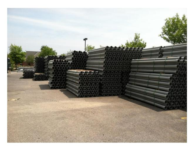
The conduit bank uses a LOT of plastic pipe – 20 miles or so, by the time the project is complete. Excavators dig a trench, then crews carefully install the pipes. A form is built around it, and then the conduits are embedded in concrete before backfilling. You may have noticed manhole structures along the way, too. Once the conduit bank is completed, utility companies will pull their lines through the conduits.
