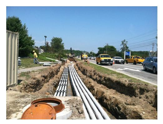
This view from August 5 shows the duct bank installation as it heads north. The photo was shot across the street from Bath Savings. A utilities manhole with emerging conduits can be seen in the foreground. Electrical conduits are shown on the right side, running up to an electrical structure. Just beyond this area, an excavator is cutting the trench for an extension. Up to 200' of installation per day is possible.
