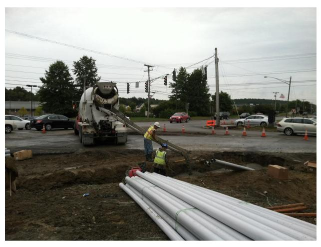
This image, taken Tuesday, September 16, shows a crew from Moulison North at the northeast corner of the Bucknam Road/Route One intersection, in front of Norway Savings Bank. This is duct bank work. We see several conduits rising above ground, and we see a concrete pour under way that will encase other conduits continuing north. The worker standing in the trench is passing a vibrating tool through the wet concrete to ensure that voids are eliminated from the pour.
