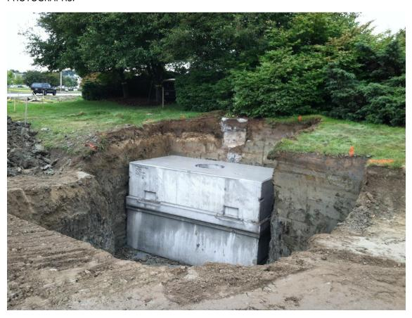
We're looking south at the southwest corner of the Bucknam Road/Route One intersection, just north of the Irving convenience store. This is one of two utility manholes set today (the location of the second one is in the foreground). The manholes are delivered in two pieces - top and bottom. A layer of dense, sticky sealing tape sits between the two halves.
