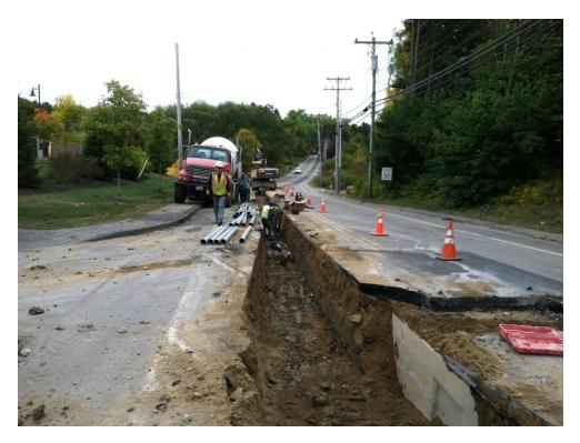
In this shot, we see crews from Moulison North installing the last section of duct bank leading up Depot Road to the Fairpoint Building. This installation is nearly complete, and re-paving of the duct bank trench on Depot Road is expected to start on Wednesday. That's a manhole structure in the lower right of the frame.
