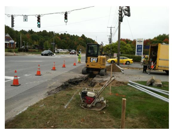
We're looking north from the northern entrance to the Shopping Plaza, directly across from Bucknam Road. This crew is excavating a trench that will contain wiring for traffic signals at this intersection.
