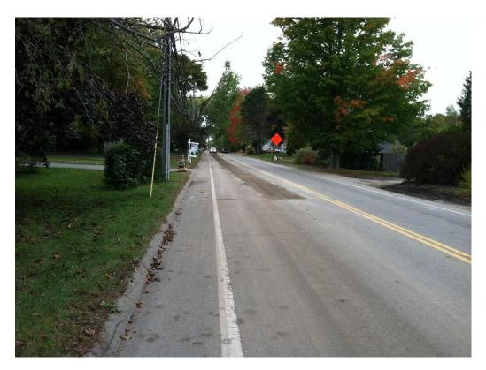
This shot looks west on Depot Road, taken from in front of the Fairpoint building. You can see the compacted backfill of the duct bank trench, which is scheduled for paving on Wednesday.
