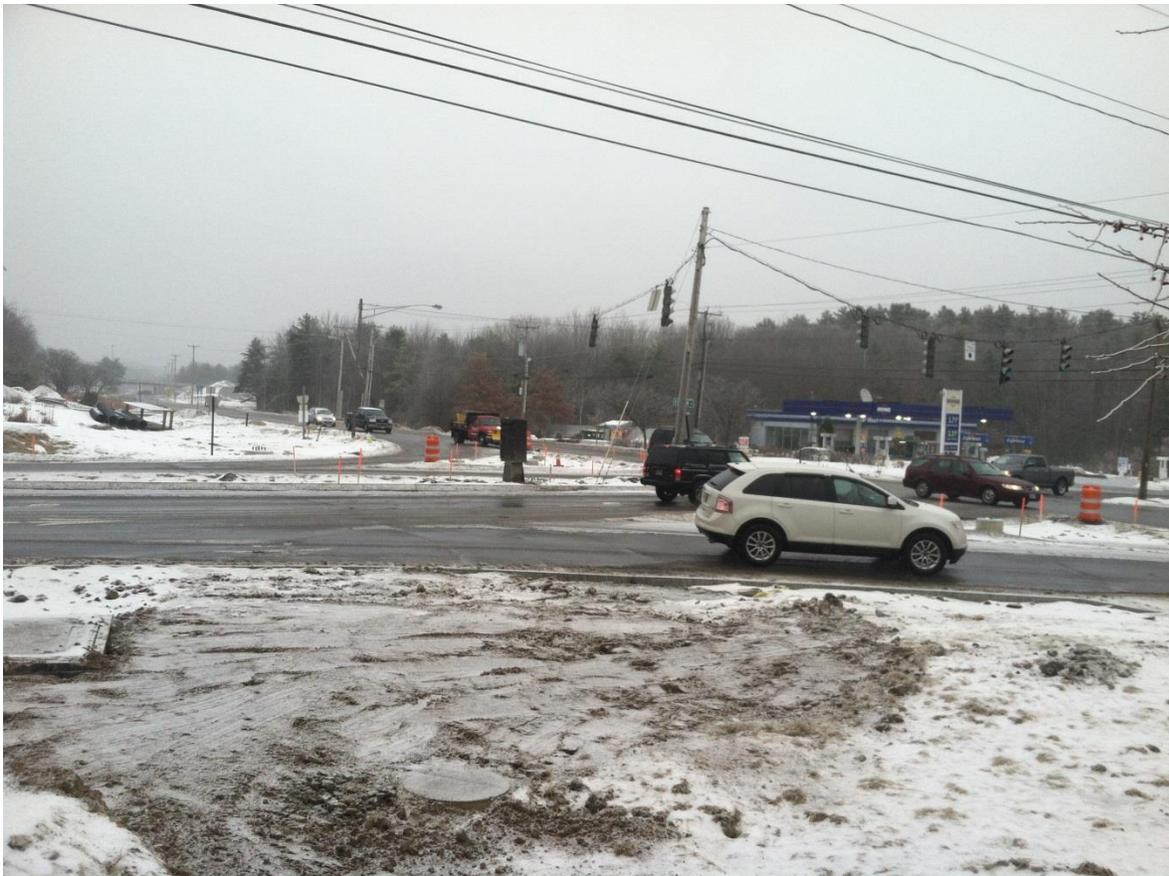
Here's the Bucknam Road intersection, looking northeast from in front of the Irving convenience store. The islands and road edges have been curbed. Stakes and barrels are in place to guide plow operators and cover bases for pedestrian lighting and signals.
