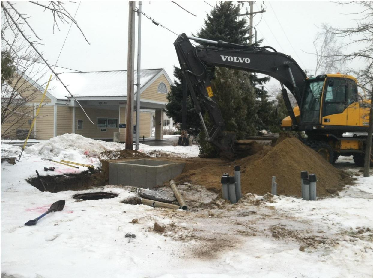
This is the final piece of major work by Moulison North – a spur of the duct bank (that’s the Bath Savings Institution in the background). Once this work is completed, Moulison has a few manholes to raise and a small amount of electrical work remaining near Morong on the west side. After that? Expect cables to be pulled through the duct bank over the winter.
