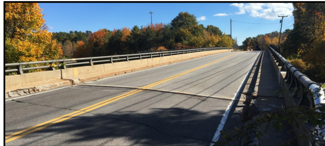
LUNT RD & BUCKNAM RD BRIDGE REHABILITATION PUBLIC MEETING
