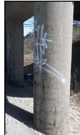
Pier 3 Cracking
