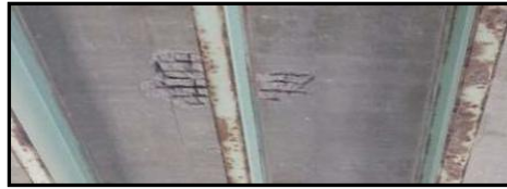
Deck Deterioration
