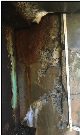
Backwall Deterioration
