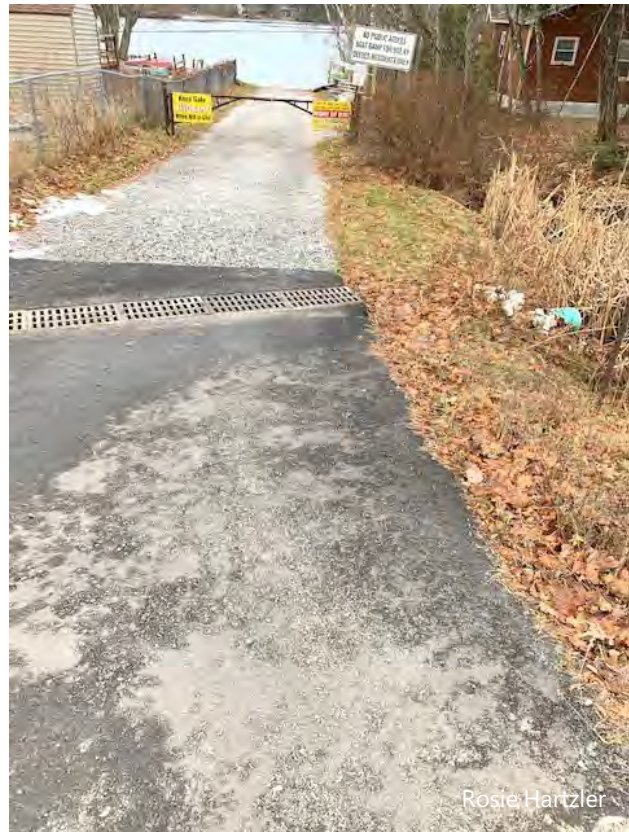
Infiltration Trench at Swan Road’s Right-of-Way
