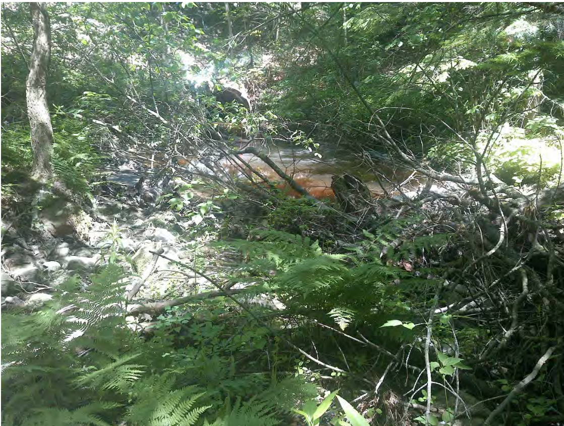
Site 1. View of debris dam looking upstream
