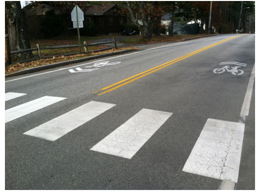
High visibility crosswalks and shared use lane markings (“sharrows”) along Yarmouth’s West Elm Street provide precedent for additional use in other “in town” locations.
