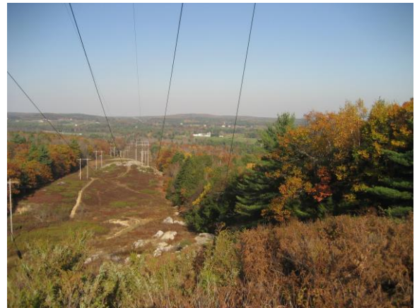
A CMP utility line bisects the property.
