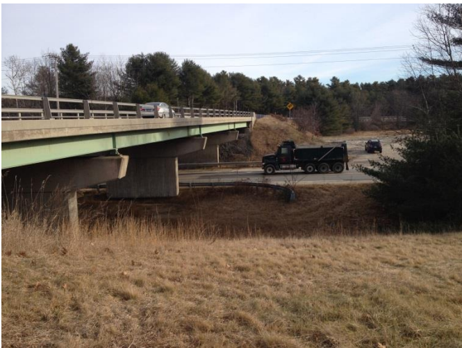
Figure 7: Bridge to be removed looking southeast
