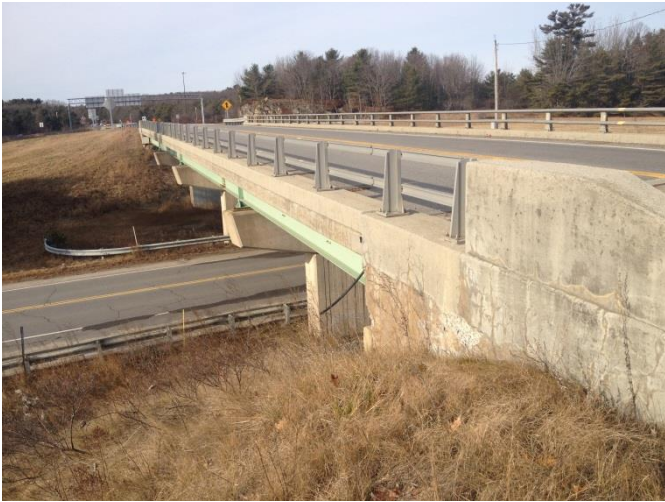
Figure 6: Bridge to be removed looking northwest
