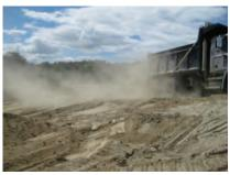
**Stabilize** all laydown areas and all unpaved surfaces with a base gravel or coarse gravel as soon as possible. Use traffic control to restrict speed and route.
