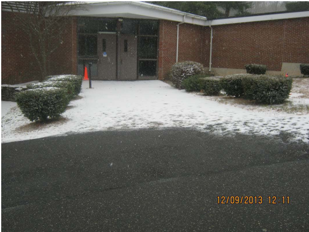
Photo 1 – Existing main entrance to the Mason-Motz building
