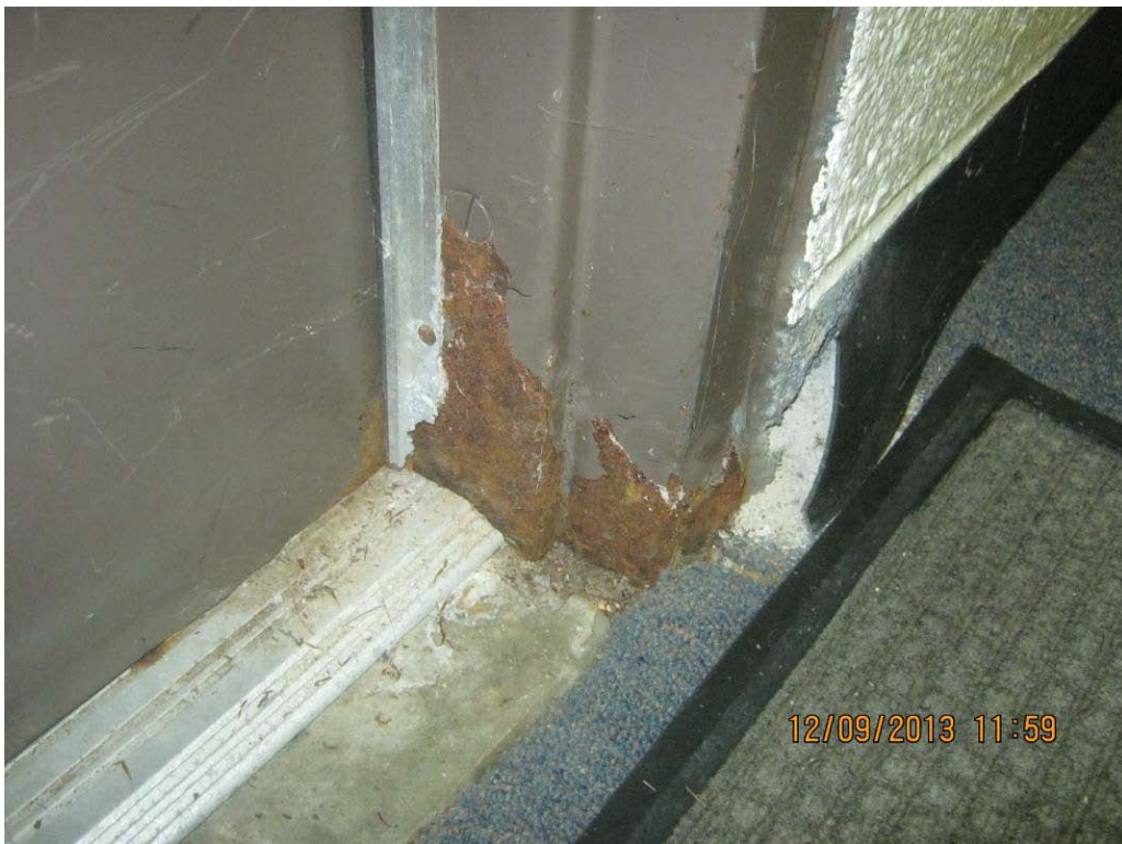
Photo 10 – Existing exterior door and frame
