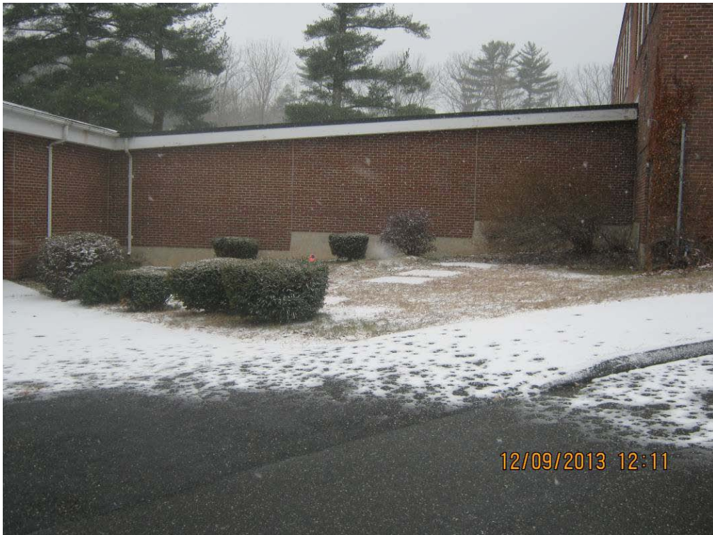
Photo 4 – Existing connector between Plummer and Motz buildings (east elevation)
