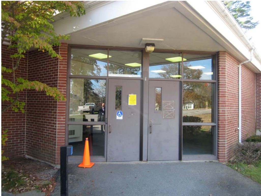
Photo 6 – Existing main entrance doors and glazing
