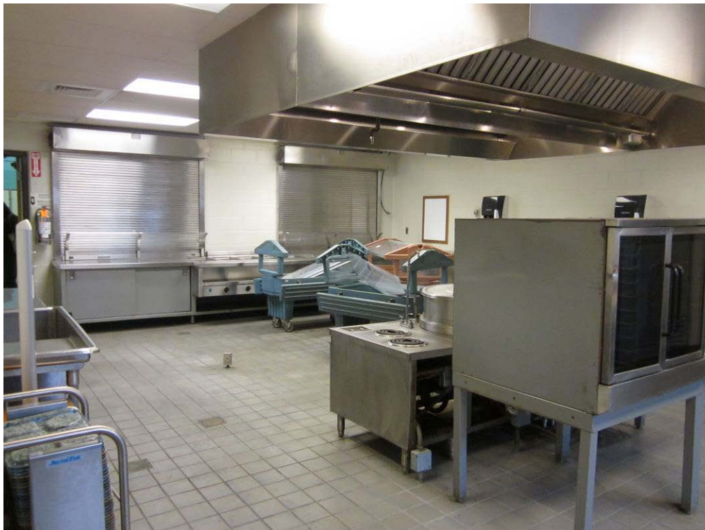
Photo 16 – Existing kitchen equipment
