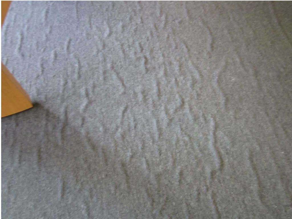
Photo 19 – Existing classroom carpet flooring
