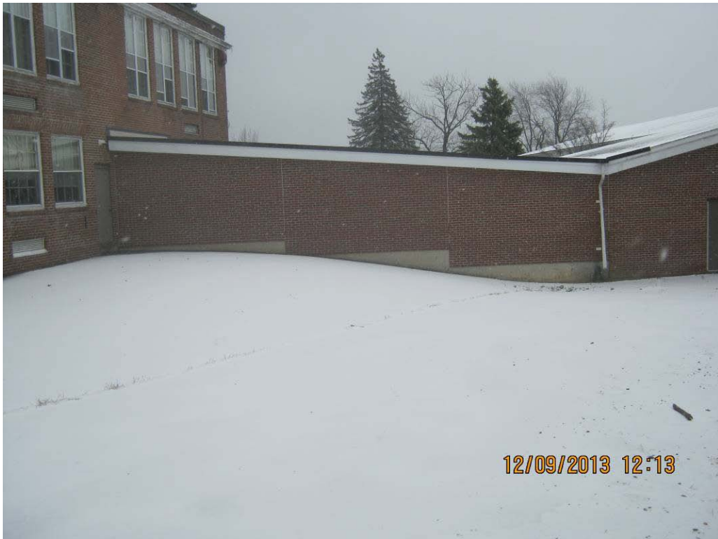
Photo 5 – Existing connector between Plummer and Motz buildings (west elevation)
