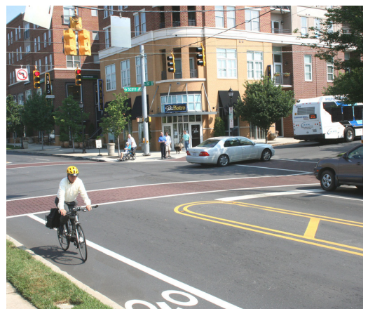
This downtown intersection features a bike lane, highly visible crosswalks and ADA-compliant sidewalks that are friendly to wheelchair users. (Photo credit: City of Charlotte DOT via Complete Streets Coalition)
