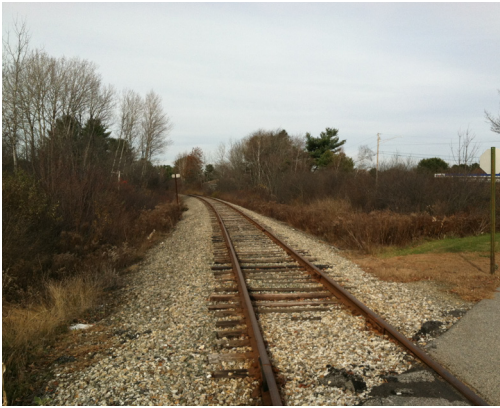
This section of the Atlantic & St. Lawrence Railway could one day feature a shared use path.
