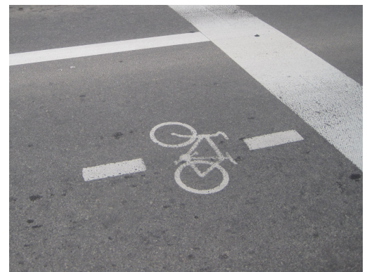
These markings indicate the presence of in-pavement loop detectors that trigger a green light when a bicyclist places their bicycle nearby.
