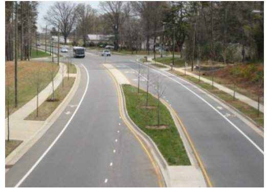
This roadway includes bike lanes so that cyclists can ride safely. The raised median in the center provides for landscaping opportunities and gives pedestrians crossing the multi-lane road a safe place to wait in the middle. (Photo credit: Flickr, Complete Streets Coalition)
