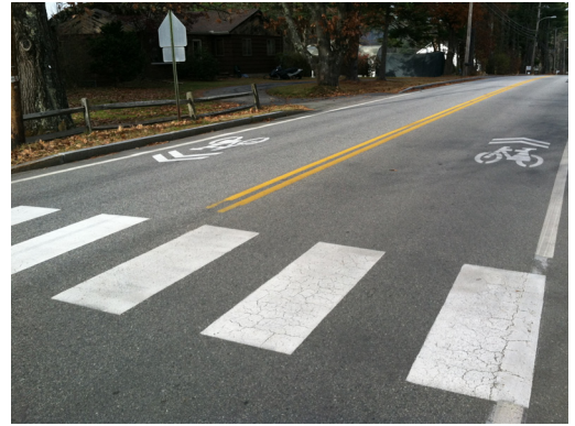
High visibility crosswalks and shared lane markings (“SLMs”) along Yarmouth’s West Elm Street provide precedent for additional use in other “in town” locations.
