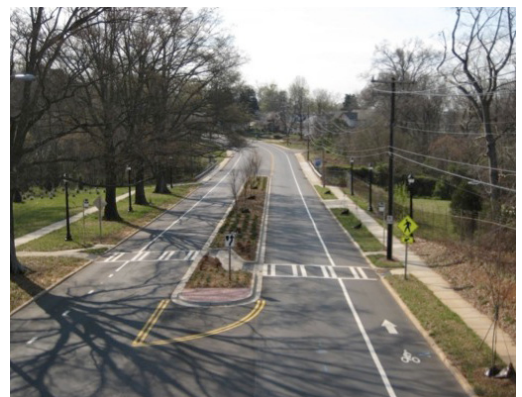
This complete street features a landscaped pedestrian refuge median with wide, well-marked crosswalks. Sidewalks and bike lanes make for safe and easy travel by bike or on foot. (Photo credit: Flickr, Complete Streets Coalition)
