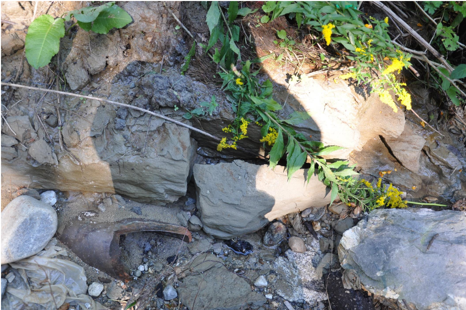
SITE PHOTOGRAPH – CHANNEL BOTTOM
