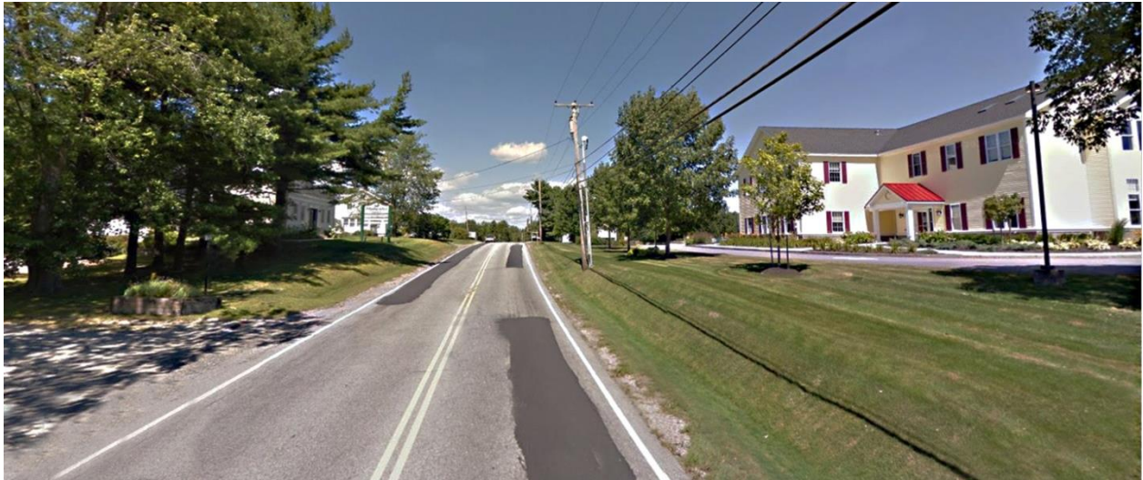
Existing view of Route 100 looking north. Cumberland County Credit Union is located on right.
