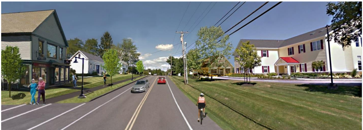
Potential future view looking north showing infrastructure improvements and hypothetical new infill development.
