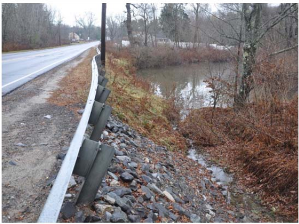
Piscataqua River south of Libby Bridge
