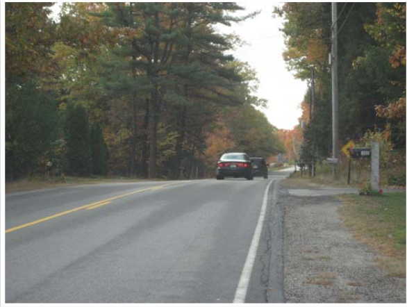
Typical road condition
