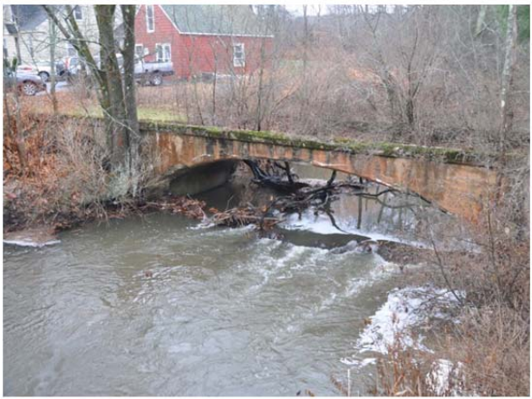
Old Portland-Lewiston Rail Bridge
