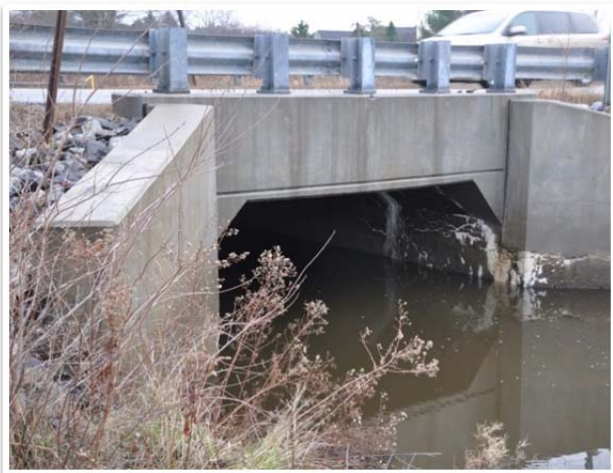
Recent bridge repairs near Cumberland Line – Piscataqua River Bridge
