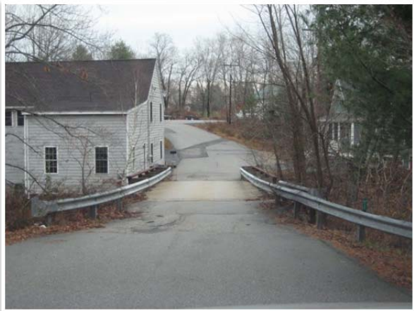
Mill Road - Piscataqua River Bridge
