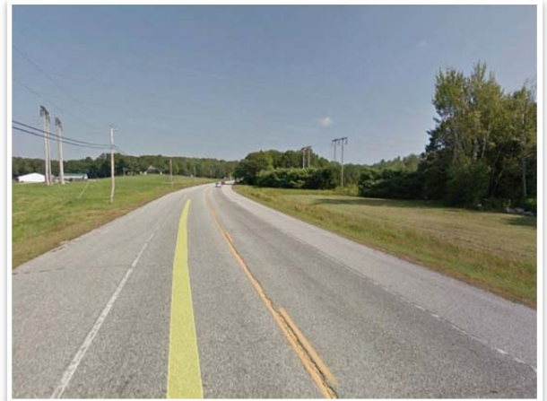
Looking north after Libby Bridge
