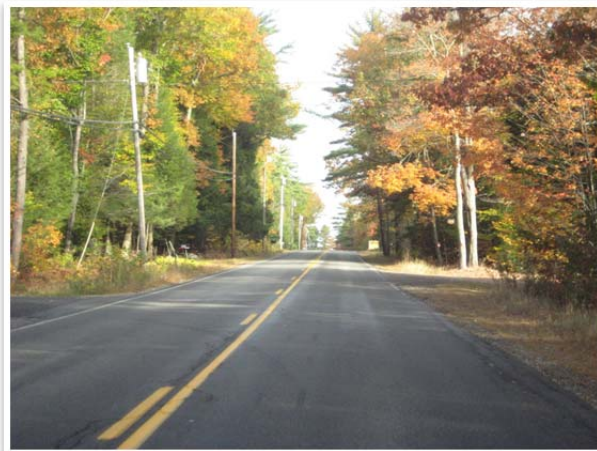
Typical road condition
