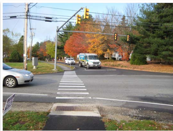
Looking west - Route 100/Leighton Road
