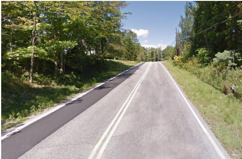
Existing View looking north, approaching Mill Road on right
