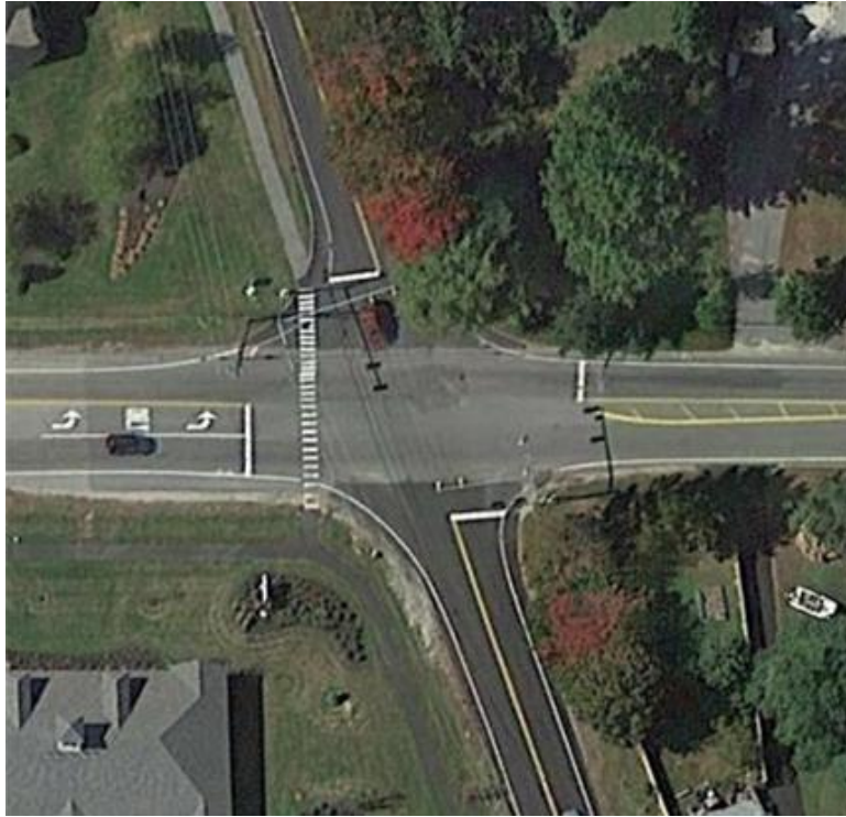
Existing Conditions at Leighton Road intersection
