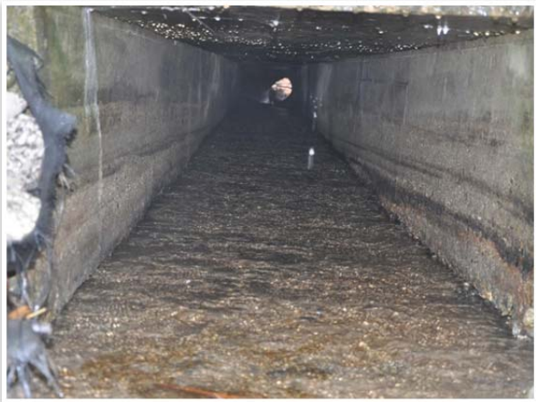
Culvert under Route 100 near Marston St.
