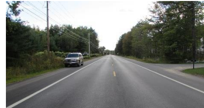
View of Route 1 North Looking South at Town Line
