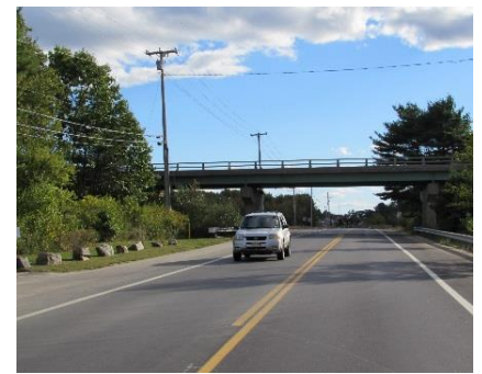
Route 1 at Falmouth Spur
