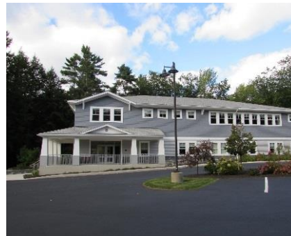
Northbrook Office Building
