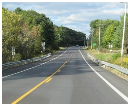
Route 1 Looking North at Sullivan Tire
