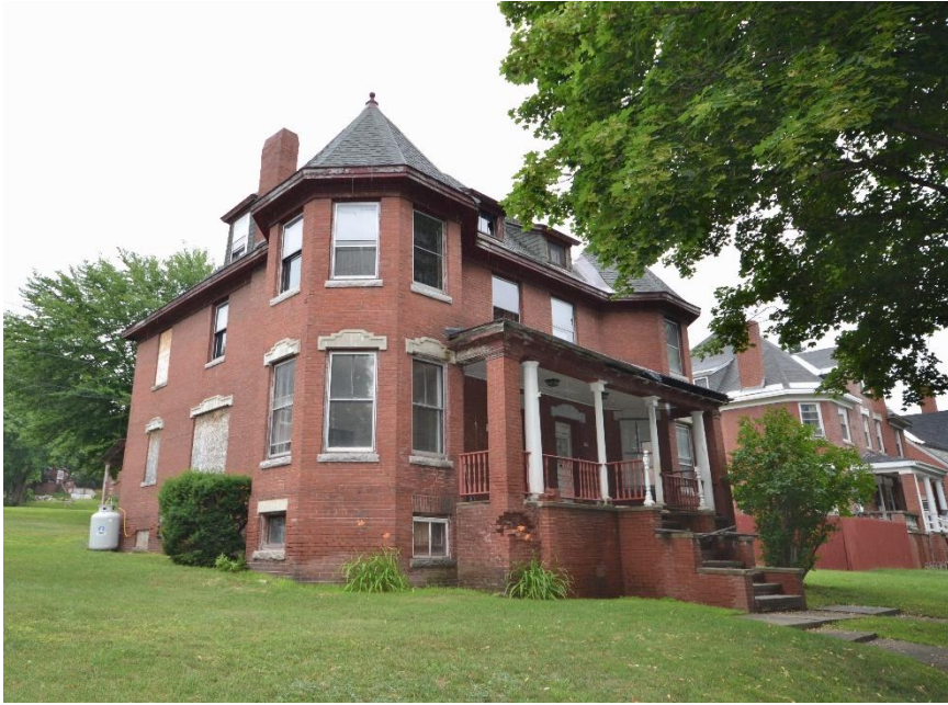
25-27 Erchles Street, Strathglass Park Rumford, c. 1903
